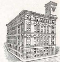
Branch collar factory, Jay Street, Troy, N. Y.
